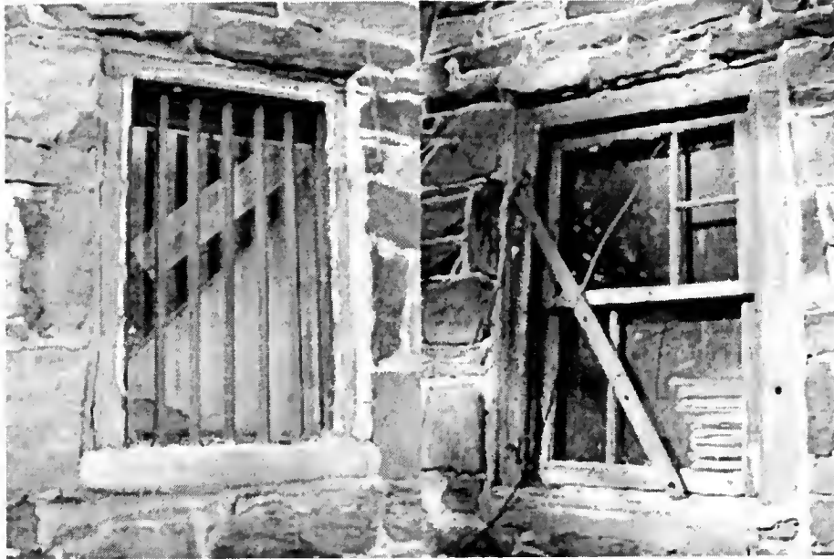
Figure 29 Window Types on Caretaker's Cottage, 2002
